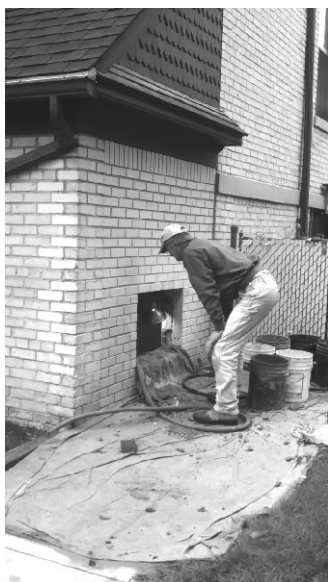
Removing the concrete steps from the old entryway to make way for the new electrical panel.
